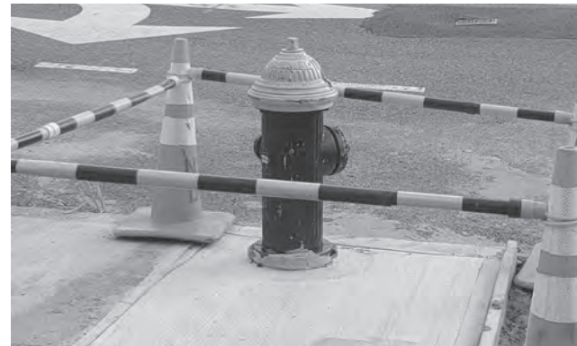
New fire hydrant standing where weeds once stood.
