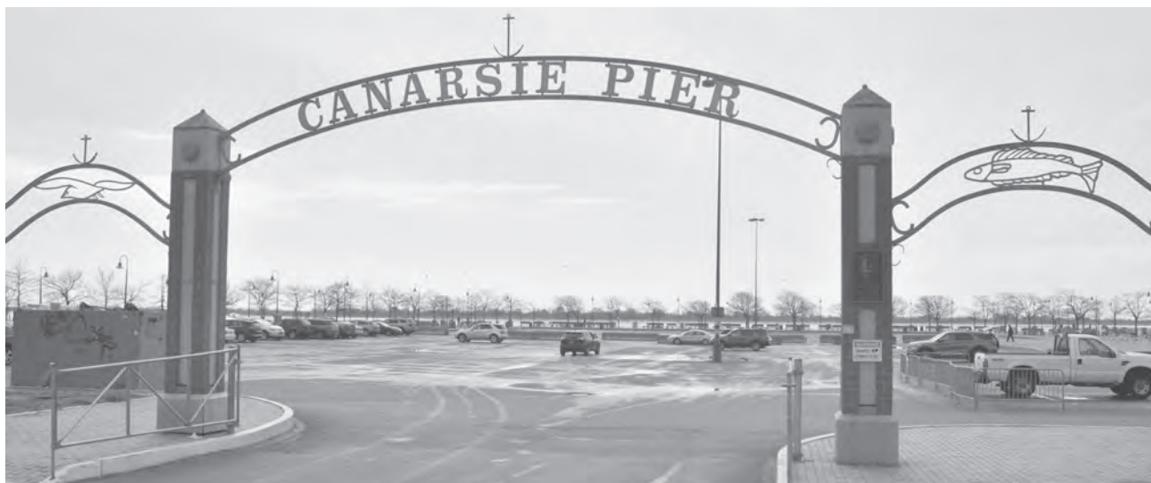
Canarsie regularly struggles with flooding, houses sinking and water leaks.
