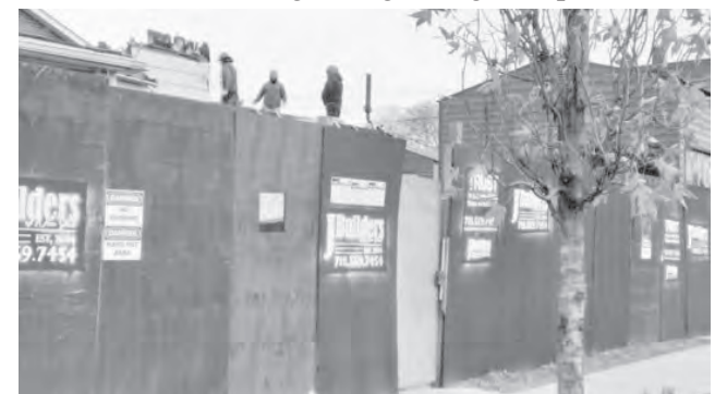
Workers demolishing the Seddio House on December 4, 2024. Photo by Linda Steinmuller
