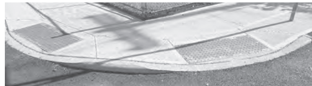
A recently installed detectable warning surface on East 91st Street and Avenue J.
